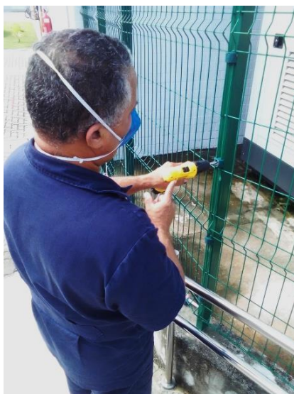
Reparo na Grade Externa
